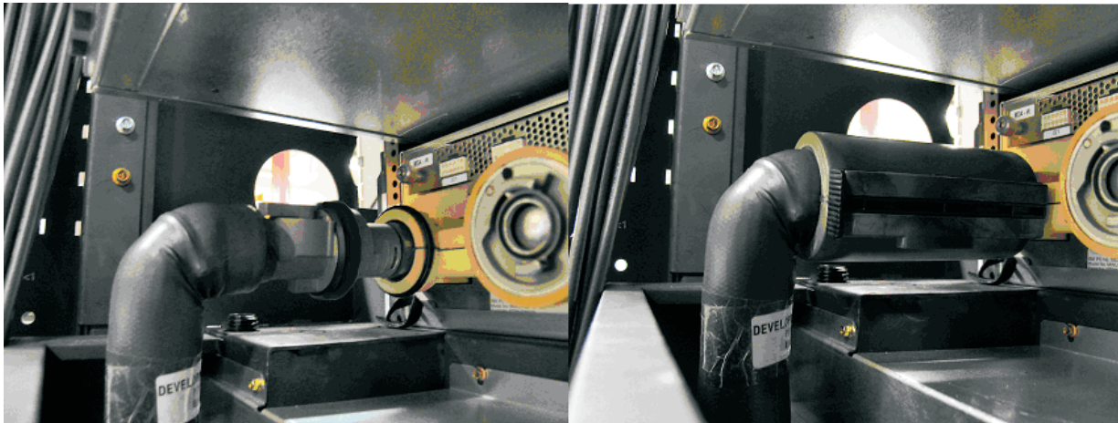
Figure 144. Quick disconnect coupling without insulator (left) and with insulator (right)
